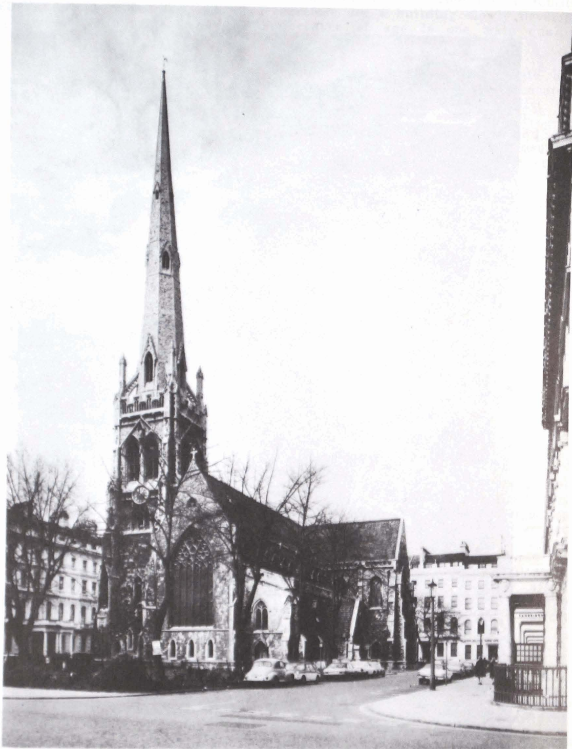
FIG. 3. Because of decayed roof timbers, Christ Church near Marble Arch, London, has now been demolished.
