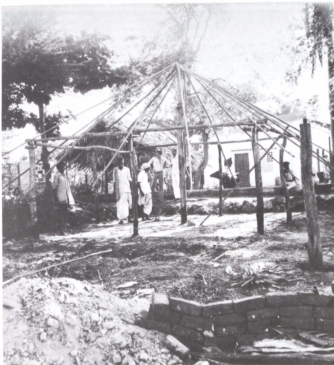
FIG. 4 - MODEL CYCLONE RESISTANT HOUSE IN ANDHRA PRADESH DURING CONSTRUCTION.
