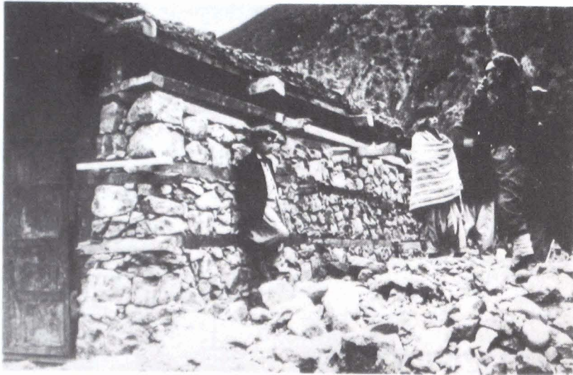
FIG. 5. Detail of method of construction used for houses near Pattan, NWF Province Pakistan: timber coursing and cross-ties, roof independently supported. (18)
